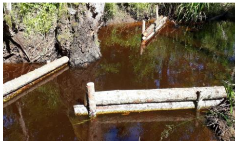
River structures built into Pudasoo river to make the environment more suitable for FPM.
